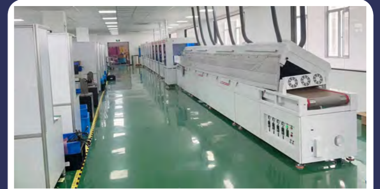
控制器车间 | Controller Workshop
